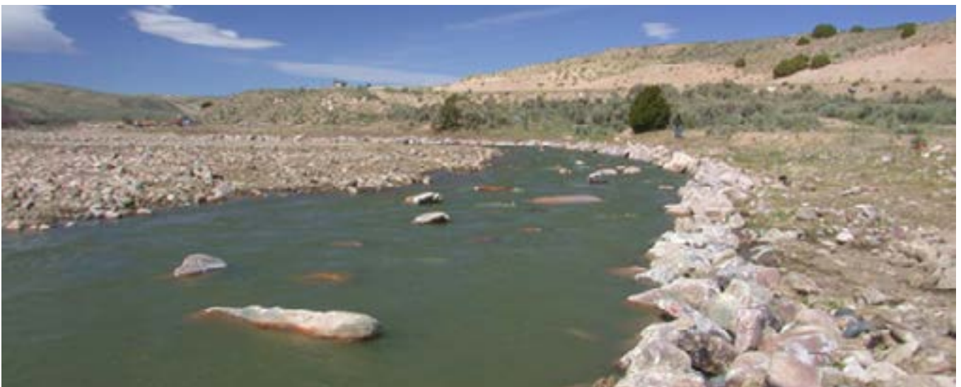
Here are two photos from Travis Cundy of the constructed 75 cfs channel. The top image from Travis is from the same vantage point as my 1999 photo. The bottom image is from a different angle. A Wyoming fishing guide calls this river reach a hidden gem of a wade fishery.
