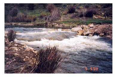
The above photo shows the same site after our work was finished. Our solution was to narrow the channel and build a permanent diversion structure. This structure really works well to divert water into the irrigation ditch...just as the gravel push-up dam did. But, more importantly, the new structure allows fish passage up or down stream at any flow, and it stabilizes the channel width.
